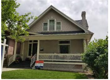
expansions. The shed dormer doesn't appear on the 1950 Sanborn Map. There is a building permit card from 1955 that includes a "bathroom remodel for dormer," which makes it likely this dormer addition dates from 1955. The 1955 dormers are also clad with wood shingles that vary slightly from those on the original gables.
